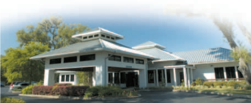
Ocala Eye Surgery Center, the newest and most advanced facility of its kind in the area.
